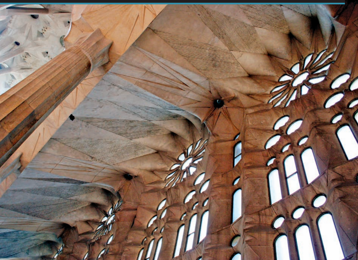
An interior view of the towers
