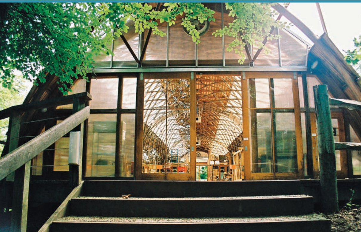
The main entrance to the Gridshell
