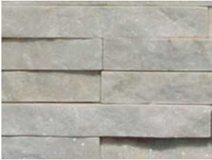
Stone wall cladding
